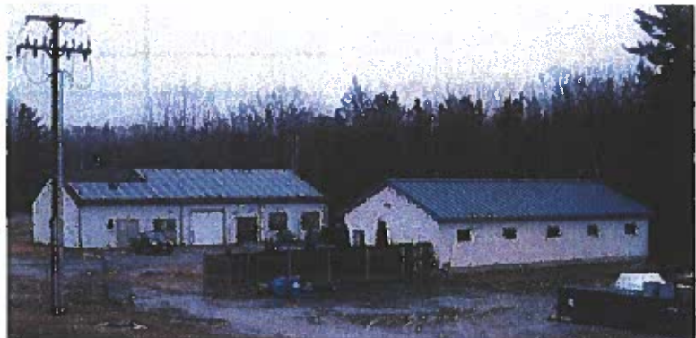
Figure 4: Control Building (background) & Garage Building
