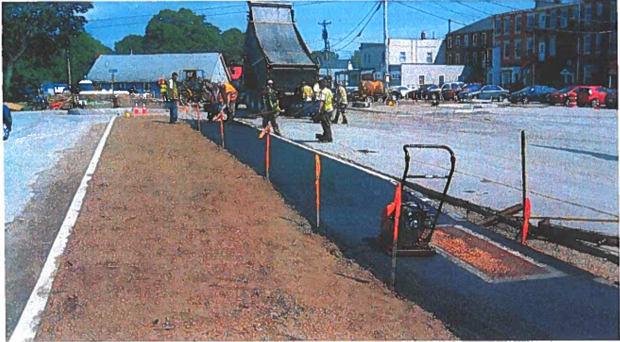
Sidewalk construction behind the Business Block in 2019
